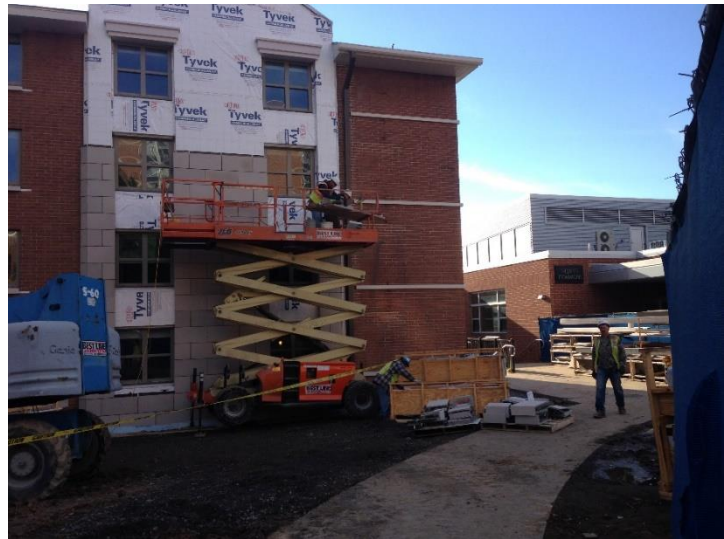
Figure 55: Installation of Limestone Panels
